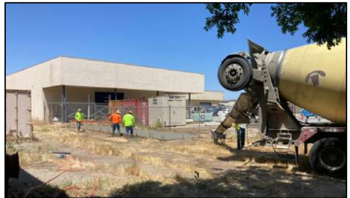
Pouring the foundation for a new container.
