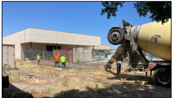
Pouring the foundation for a new container.
