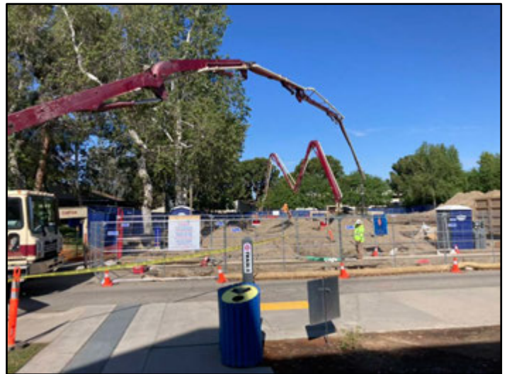
Preparing for construction of the new Energy Innovation Building on CSUB campus.
